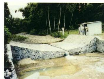
PLATE 26 A non-standard weir in Java on a stream carrying a very heavy bed load
